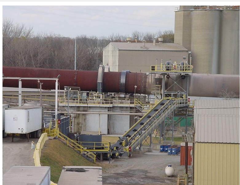
Used tires being fed to a pair of cement kilns
