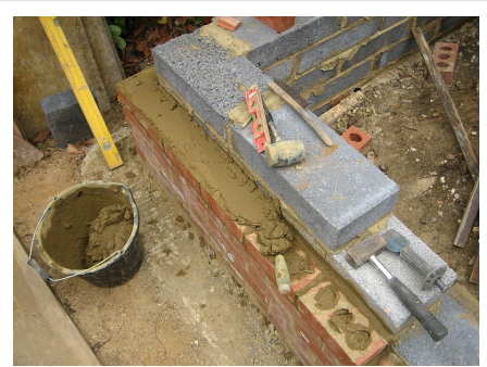
Laying bricks with portland cement mortar
