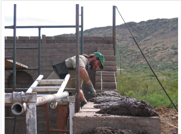
A mason laying mortar on top of a finished course of blocks, prior to placing the next course.
